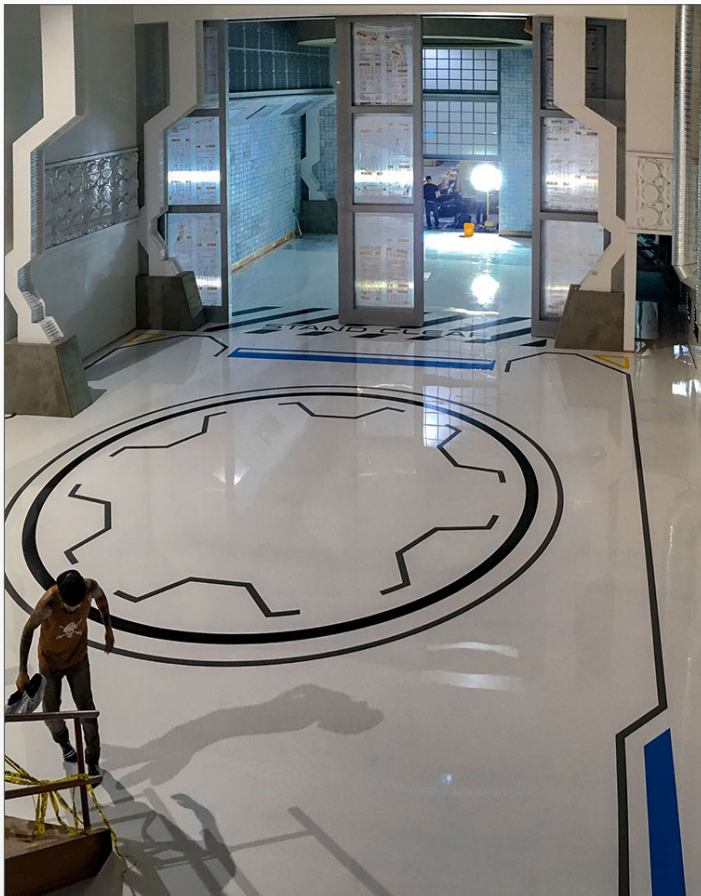
Vinyl Cut Graphics under Clear Epoxy Floor
